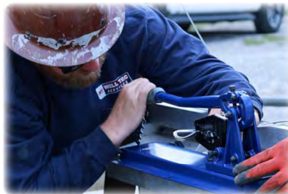
Cable Installation at the Pomona Extensometer Facility
